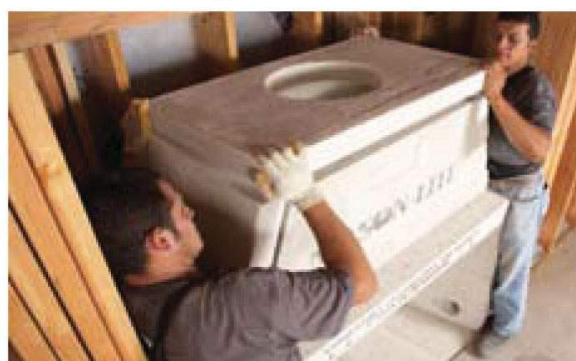
4. Finishing with the dome top
