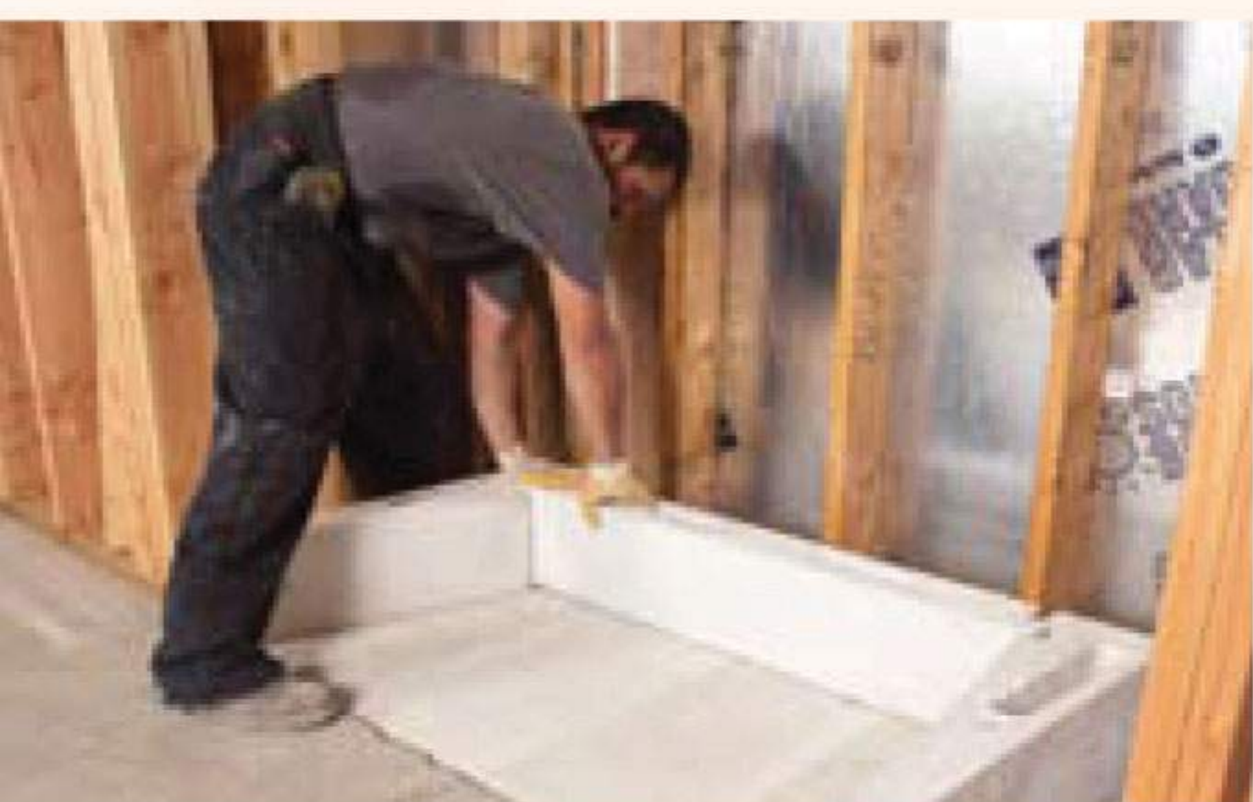
1. Installing base and first course
