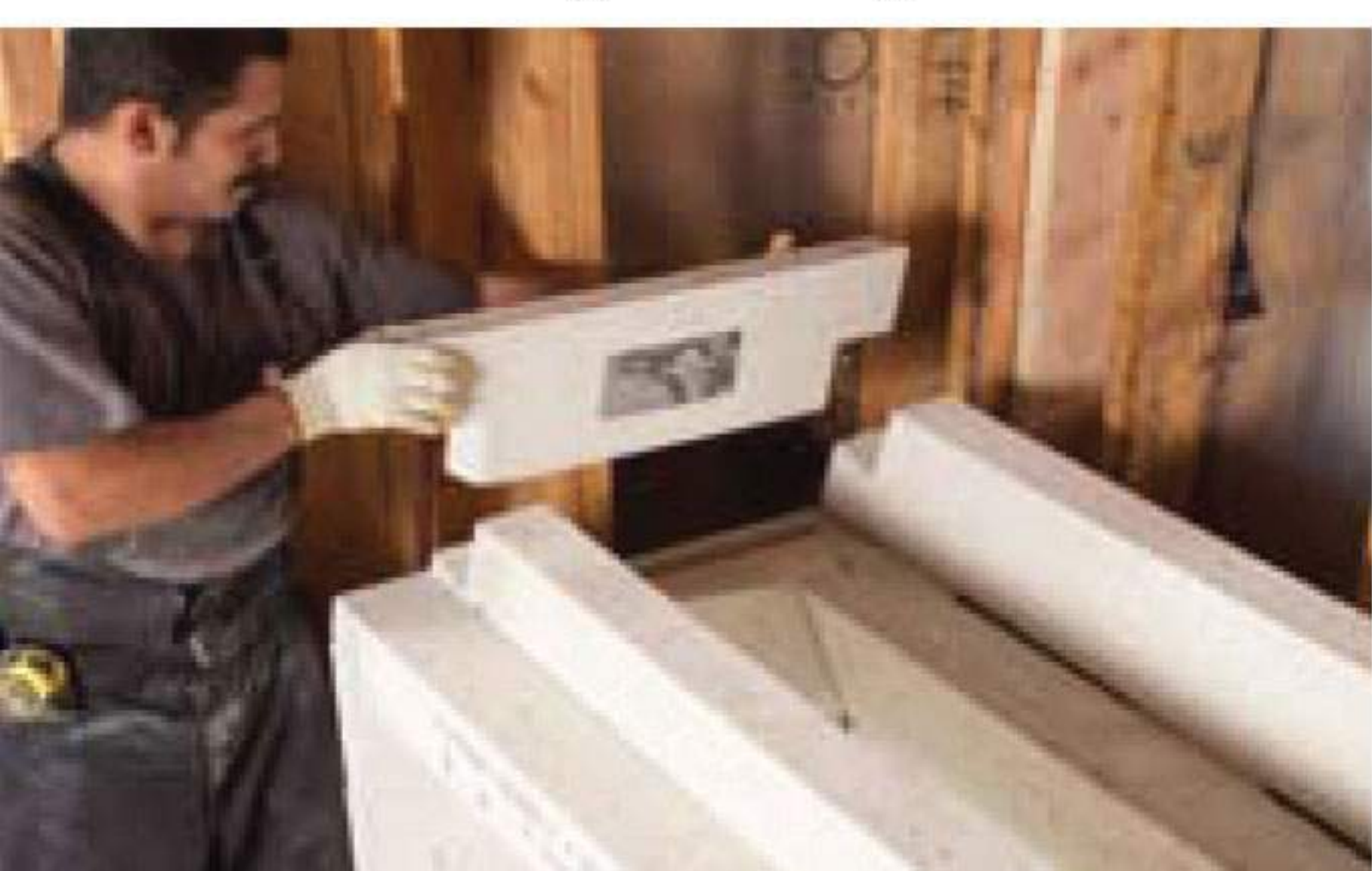
3. Easy to build smoke dome
