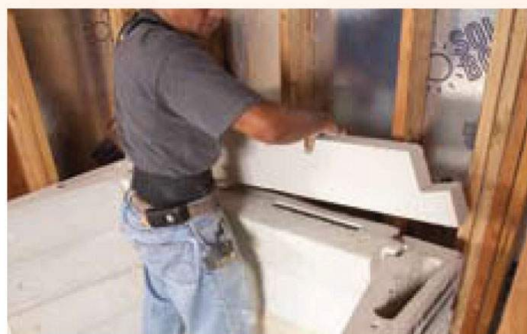
2. Starting the smoke chamber
